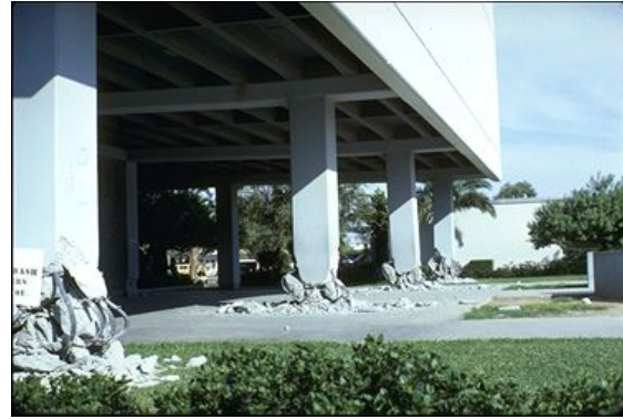
Fig. 17. Inadequate details at the base [19-23]
