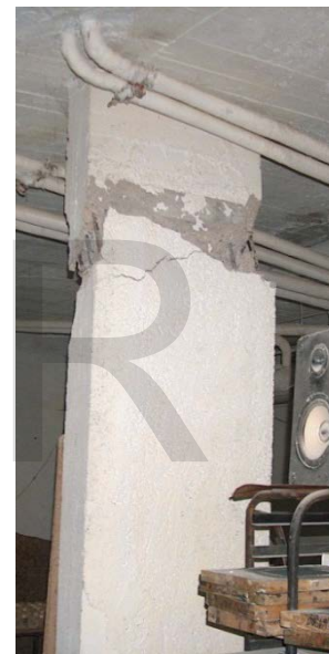
Fig. 22. Creep failure, heavily damaged column in an apartment [42]
