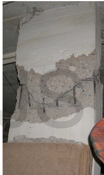
Fig. 22. Creep failure, heavily damaged column in an apartment [42]
