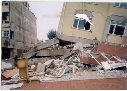
Fig. 17. Inadequate details at the base [19-23]
