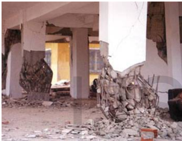
Fig. 6. Columns failure with buckled longitudinal bars
