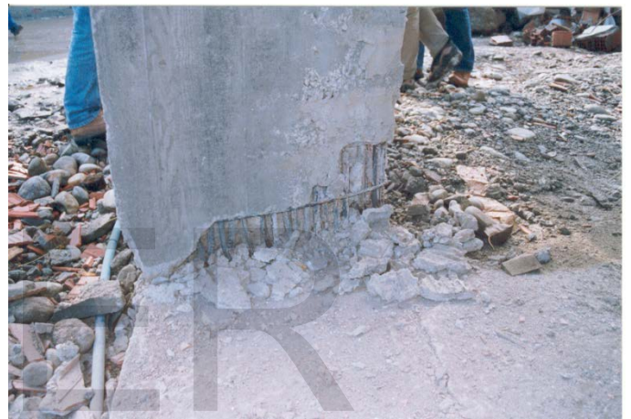
Fig. 6. Columns failure with buckled longitudinal bars
