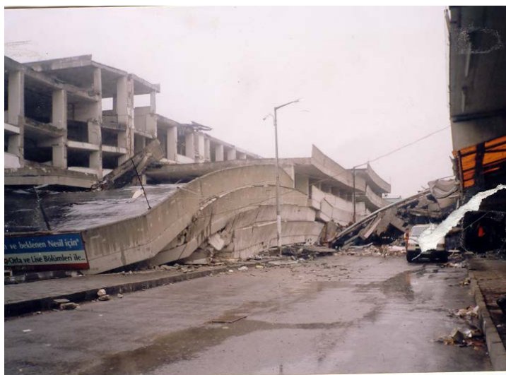
Fig. 12. Shear failure of flat-plate construction (punching failure)
