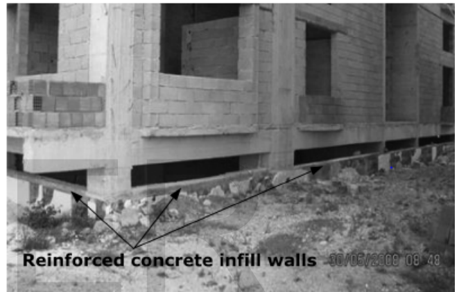
Fig.9b. Short column effect [23]
